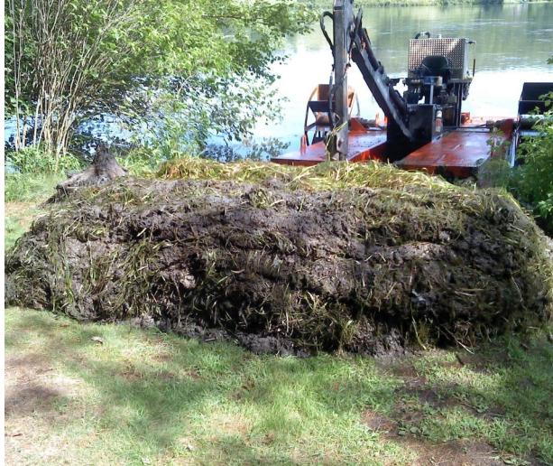
The Hydro-Rake, which is seen at the shoreline as it removes submerged aquatic vegetation, root mass and attached hydro-soils from a waterbody, creates a spoil pile which will then be moved to a dewatering or compost location to dry out away from the shoreline.
