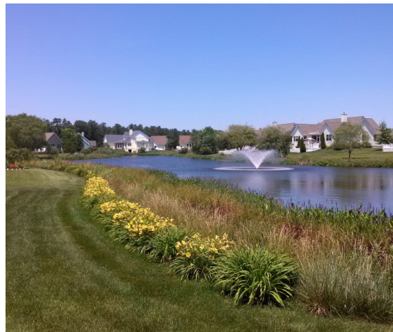
Shoreline beneficial emergent vegetation, along with properly sized aeration, either submersed or floating as shown here, are both strategies that can be employed in an Integrated Pest Management (IPM) plan for your stormwater pond.
