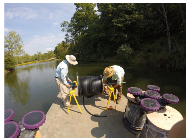
A submersed aeration system can help oxygenate the water column in deeper lakes and ponds. These systems improve vertical mixing at depths where water is not naturally stratified by using an on-shore compressor to pump oxygen to the bottom of the waterbody.
