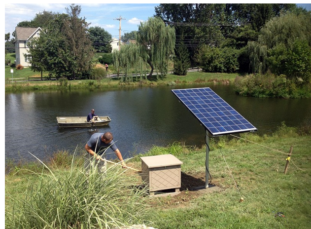
For remote locations or waterbodies without electrical power accessibility, solar powered aeration systems offer a long-term, ecologically responsible solution.
