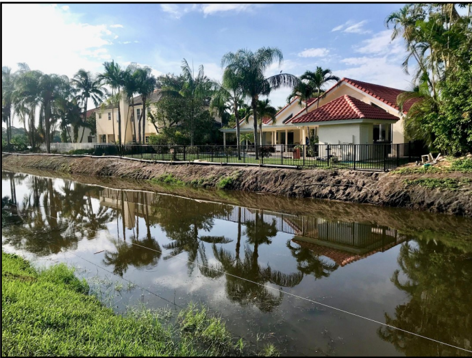
HOA Erosion Control BEFORE
