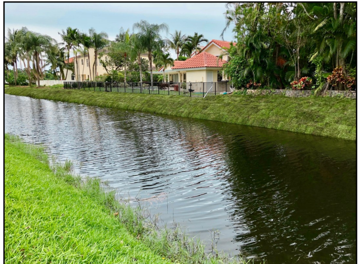
HOA Erosion Control AFTER
