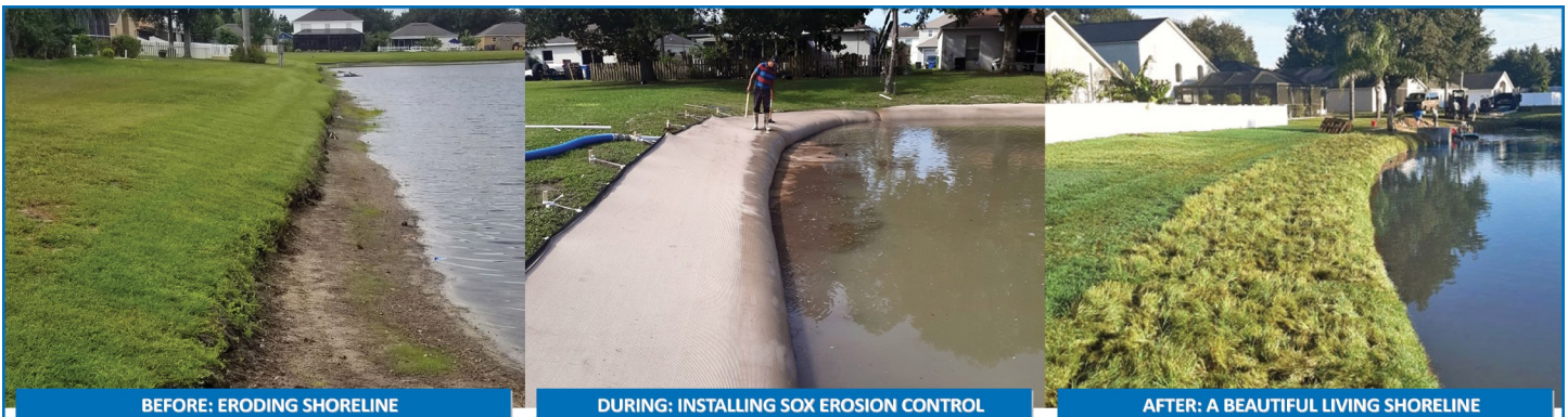
BEFORE: ERODING SHORELINE
